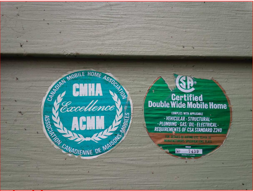
Mobile Home 100 A Main Breaker
